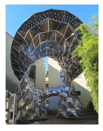
Figure 9. *Bloom* was made of 414 structural or performative panels.
